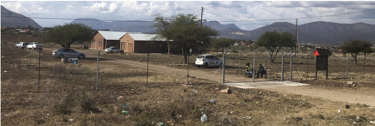
Exploration camp, new fence and manned security gate.
